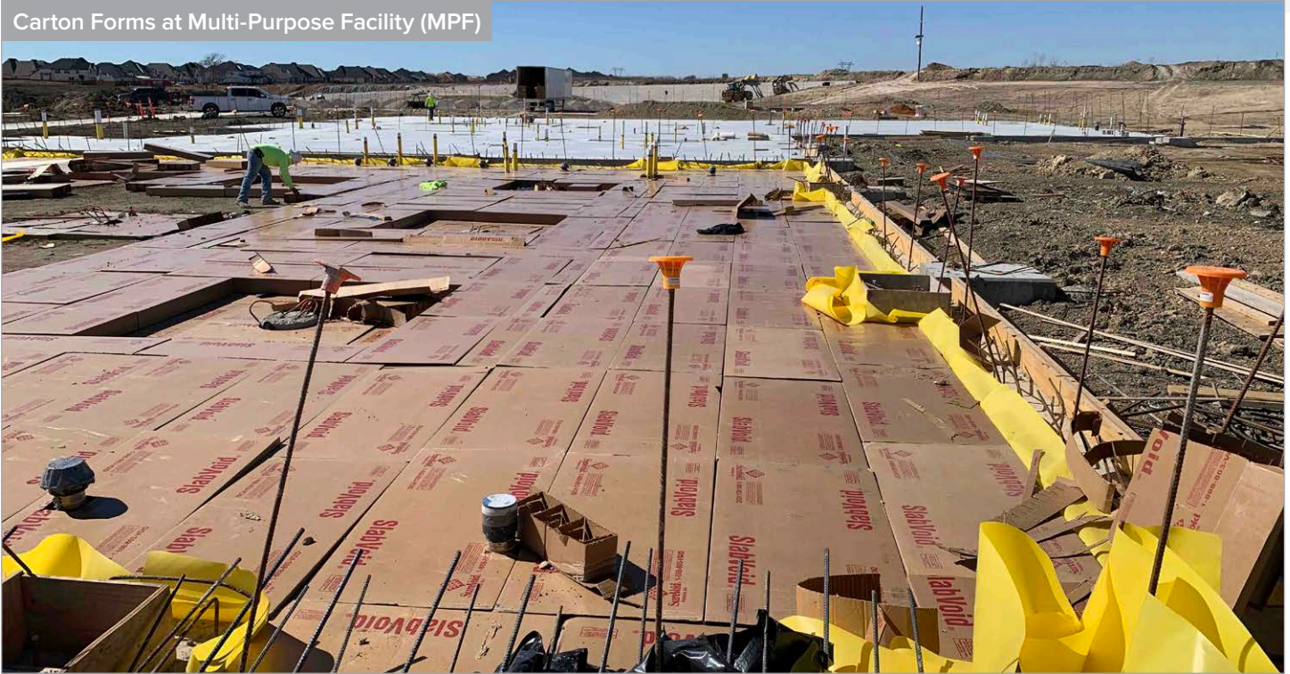
Multi-Purpose Facility (MPF) Indoor Area
